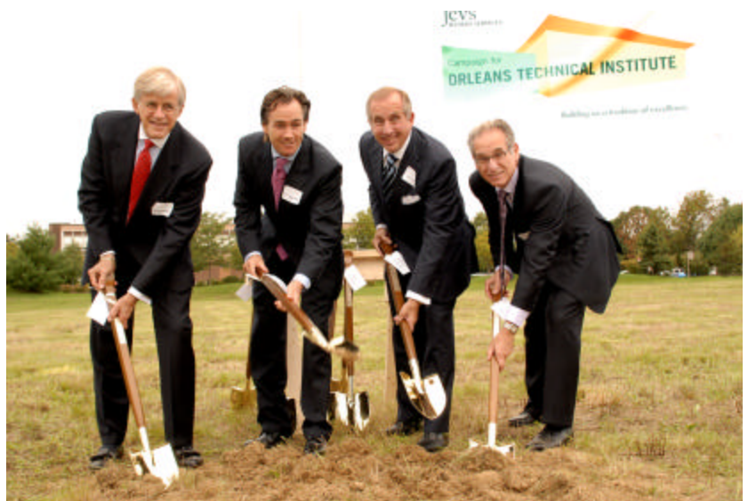
Above: JEVS Human Services Board Chairman Ben Zuckerman, State Senator Mike Stack, Project Benefactor Jeffrey Orleans and President & CEO Jay Spector break ground on the $20 million site.
